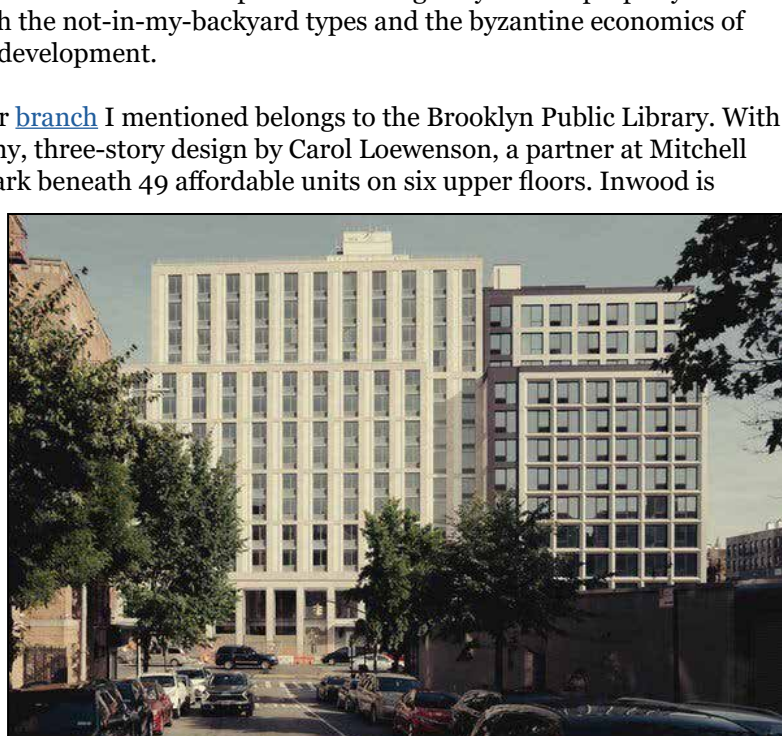
The Inwood library, left, occupies the bottom floors of a 14-story affordable housing development. Credit...Amir Hamja for The New York Times
